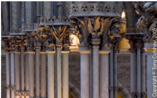
The cast iron columns supporting the glass roof in the court.
